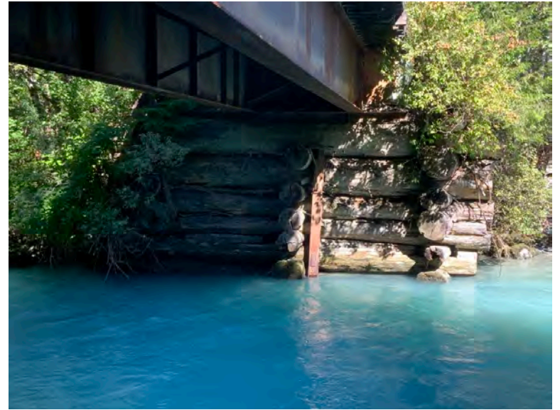
Left Bank Abutment when facing downstream
