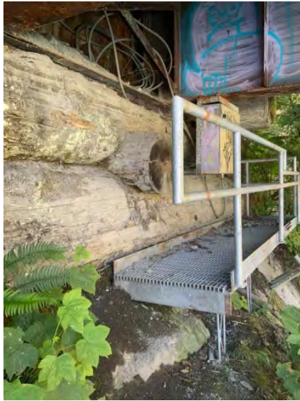
Right Bank Abutment when facing downstream
